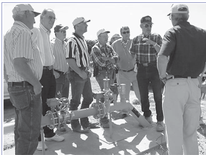
Del Church, SVID Watermaster, discusses enclosed conduit systems with SVID Board Members and staff. Pictured is a flow meter installation
