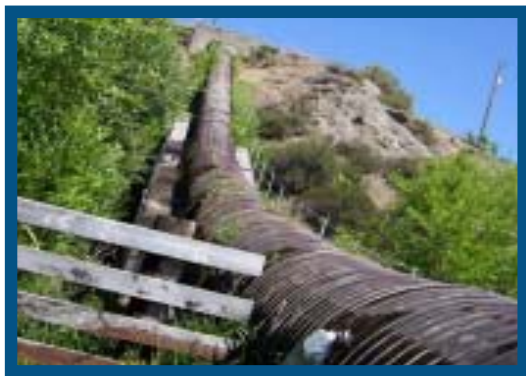
Old wood stave pipe
