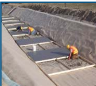
2004 concrete application to liner
