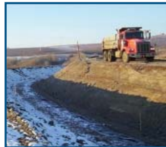
2005 Snipes Lateral 7.84 bank preparation
