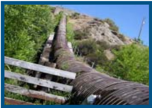
Old wood stave pipe
