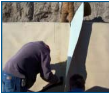
2004 gluing the liner sections
