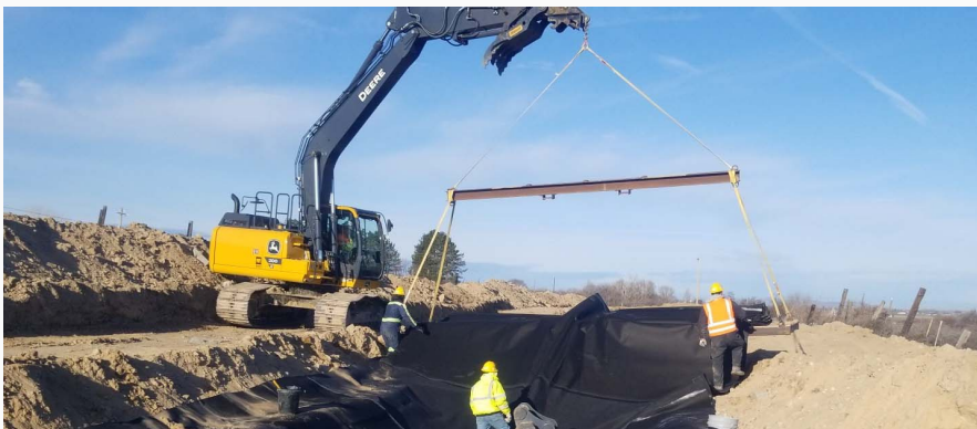
SVID Crews roll out liner in preparation for shotcrete.
