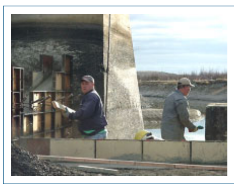
Construction has begun on Drop 1 SCADA project.
