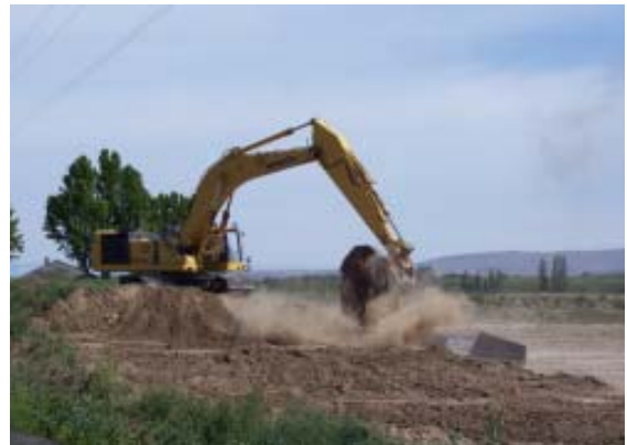
The 59.29 re-regulating reservoir on June 23, 2005.
