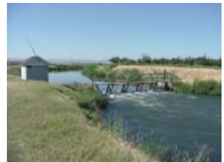
The above picture is of a manually adjusted gate that will be replaced with an automated gate.
